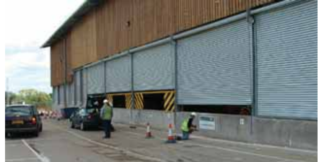
Frizlands Lane, Dagenham (London Borough of Barking & Dagenham)
