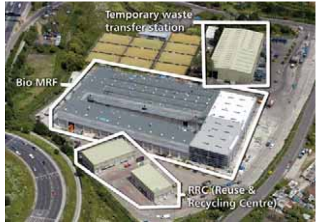
Aerial view, Jenkins Lane (London Borough of Newham)
