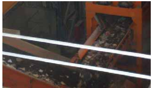
4 Residual Waste (i.e. not orange bags) being shredded
