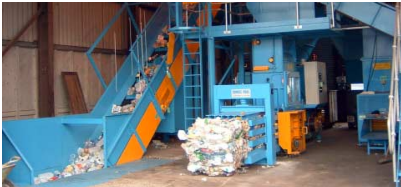
The refurbished Ilford Recycling Centre
