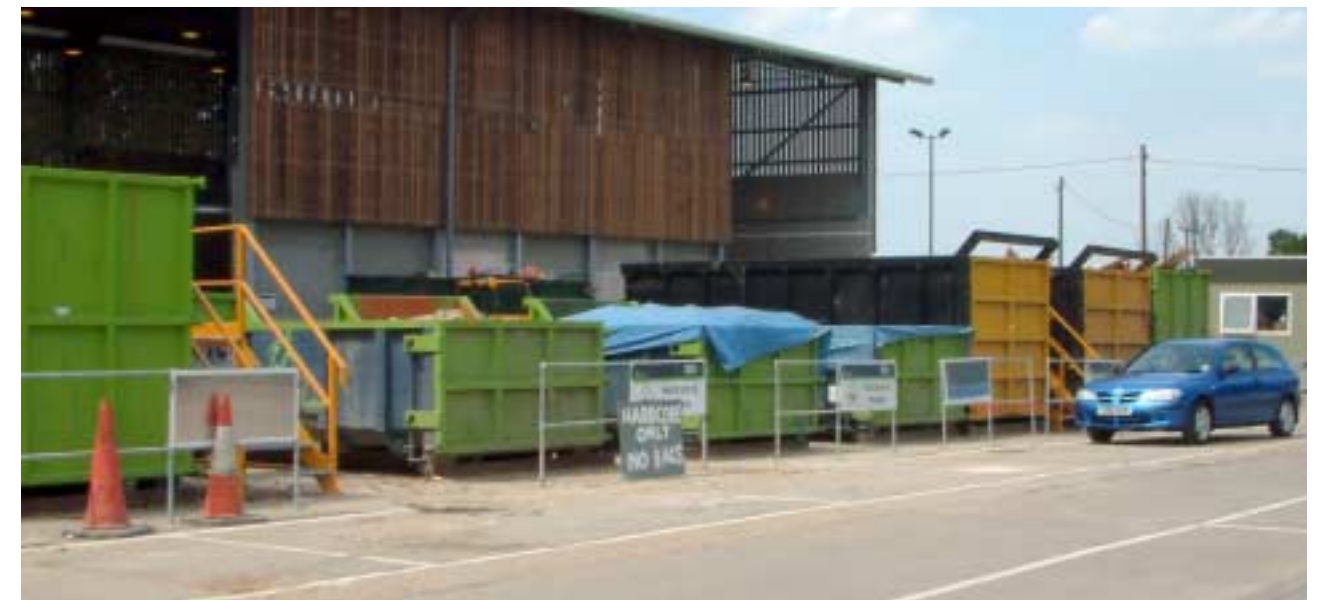
Recycling facilities at Gerpins Lane Reuse & Recycling Centre
